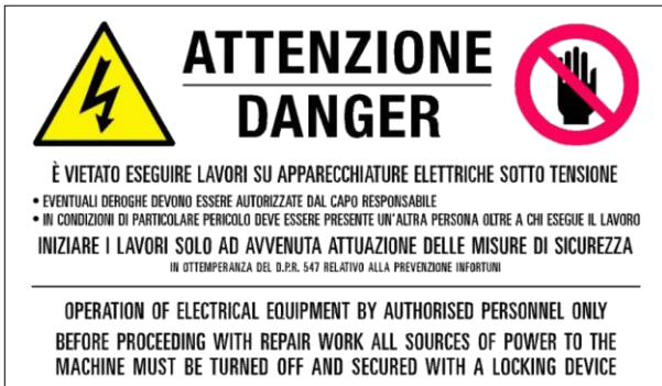
(positioned on the door of the electrical panel)
